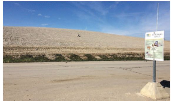
Finished slope with clay and topsoil over final HDPE cap. Ready for grass seed.
