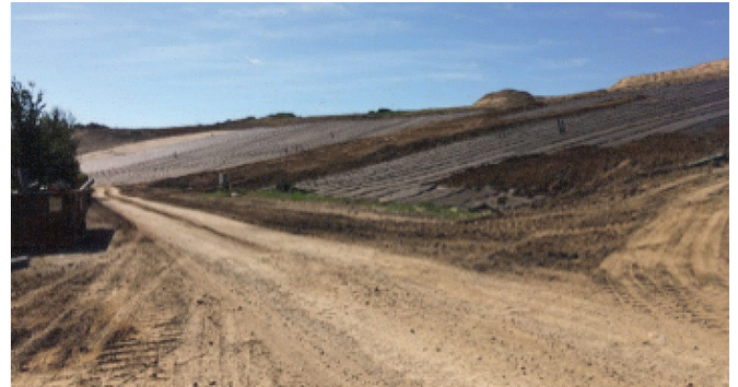
Placing clay and topsoil over HDPE final cap material.
