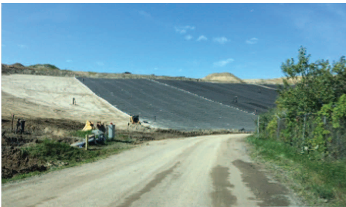
30 mil High Density Poly Ethylene (HDPE) plastic cover material in place.
